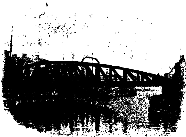
SWING BRIDGE OVER THE WEAVER.
